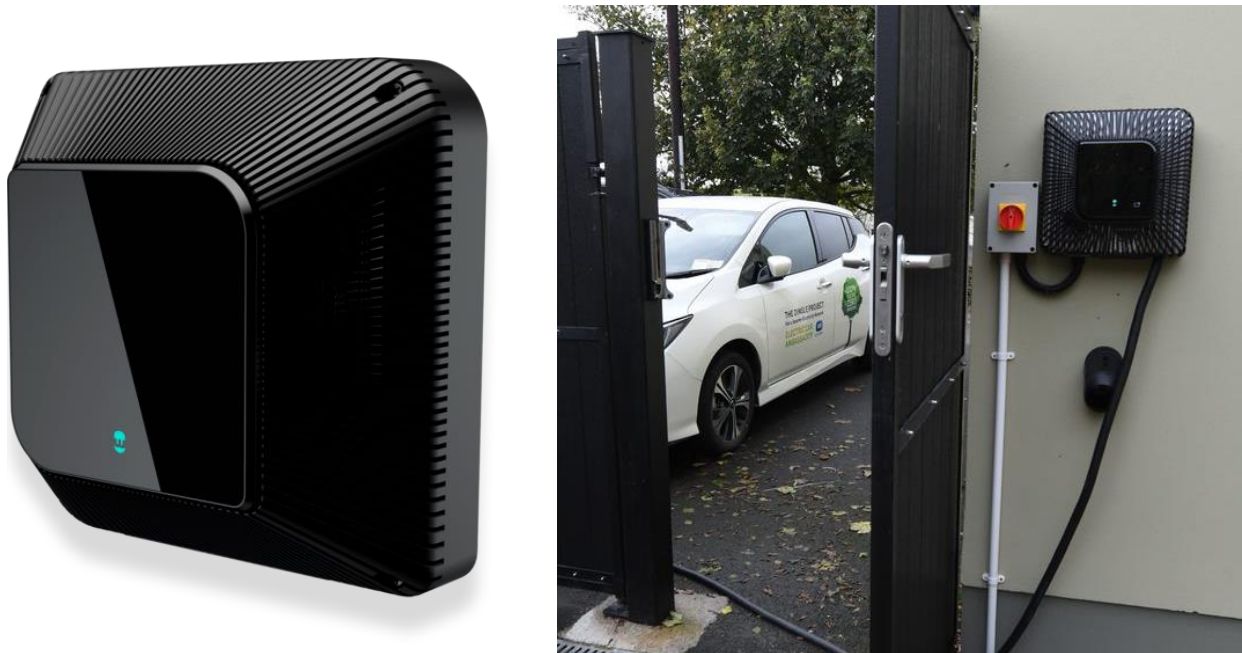
FIGURE 47 WALLBOX QUASAR VEHICLE TO GRID CHARGER INSTALLATION
