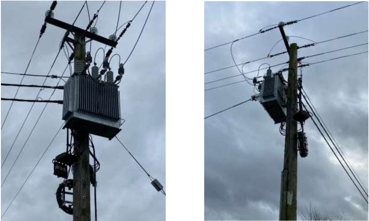
Figure 2: Pictures showing the installation of the 300 kVA pole mounted transformer
