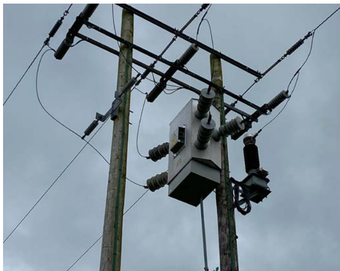
38kv remotely controlled switch
