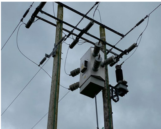
38kv remotely controlled switch
