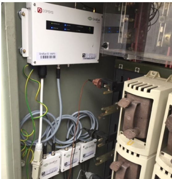
FIGURE 9 GROUND MOUNTED MONITORING DEVICE DEVELOPED BY DEPSYS
