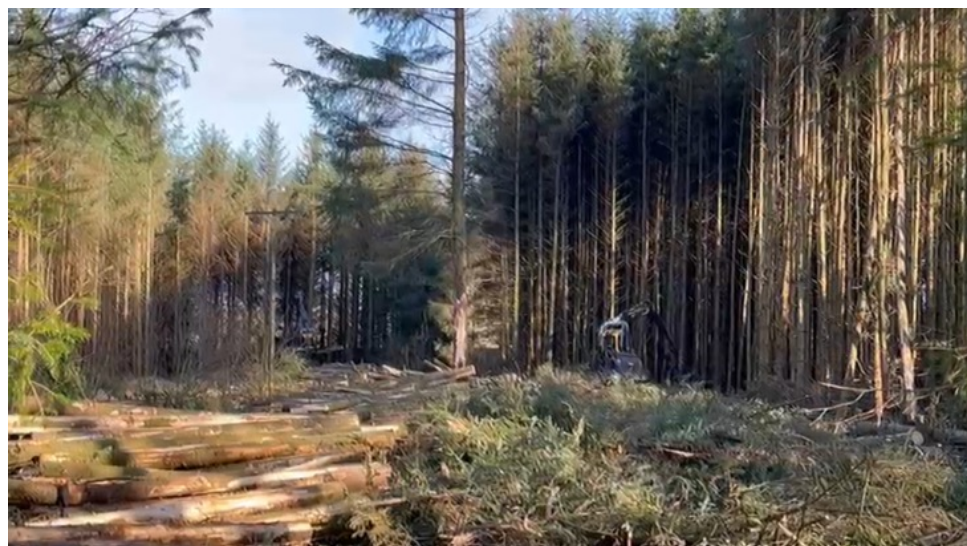
Figure 30: Sample of forestry clearing activity in Ballinlough, Co.Roscommon
