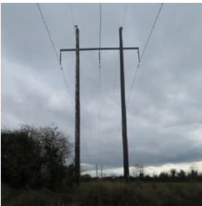
110 kV poleset with earth wire
