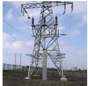
110 kV cable sealing end mast
