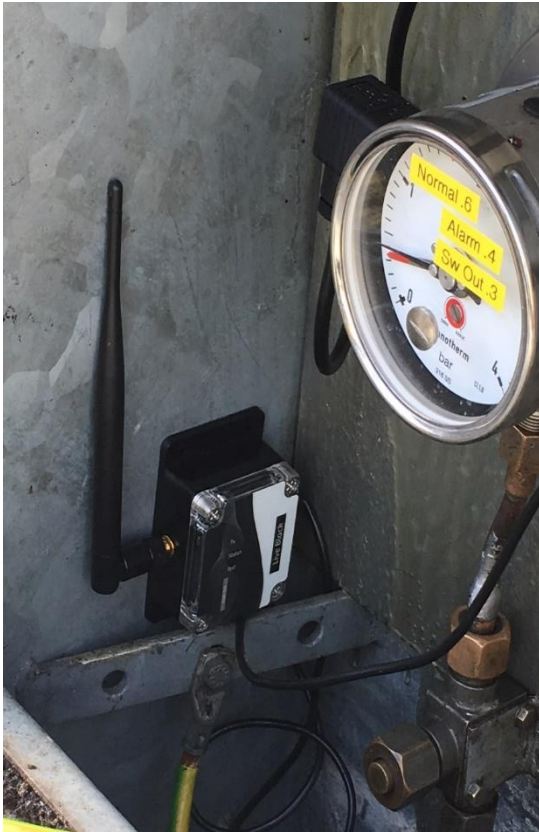
Figure 1 - Fluid Filled Cable Monitor Utilising Sigfox
