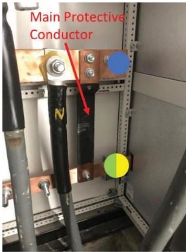
Figure 7: Example of TN-C-S in a commercial installation
