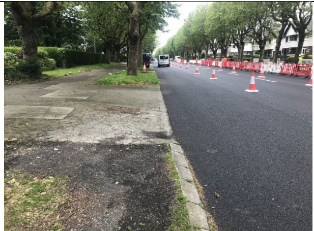
16-04 – Griffith Avenue in good condition as it is undergoing resurfacing works which are almost complete (tarmac surface).
