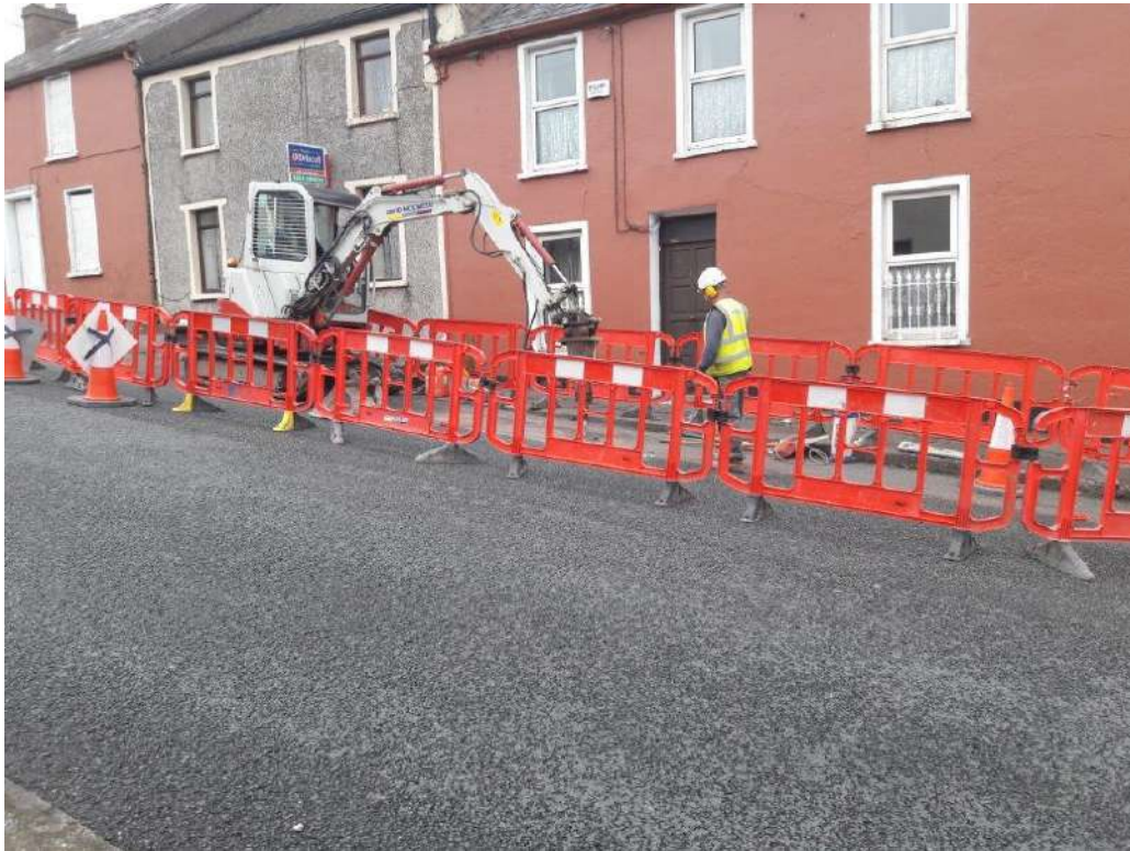
Photo 1 Cable route located on eastern side of Fair Hill.
