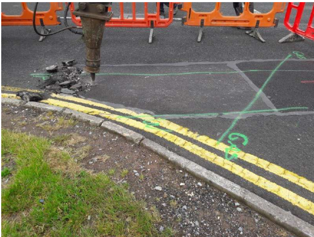
Photo 2 Location of gas and utility lines marked on road in preparation of trial pit works.
