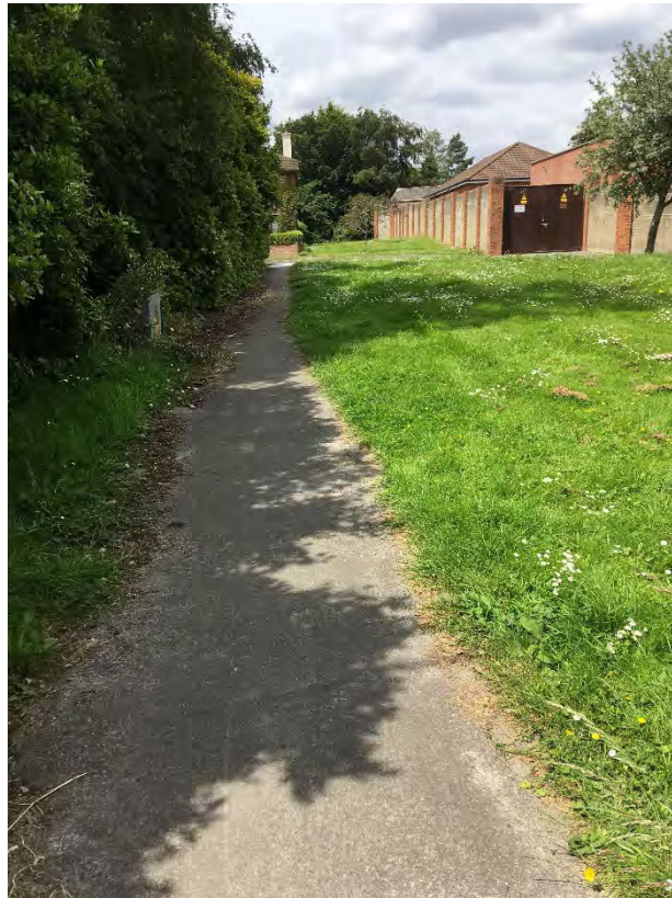
Photograph 2 – Cable route west of leak location
