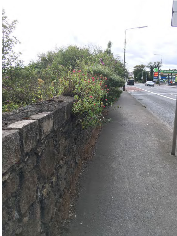
Photograph 3 – View south from leak location
