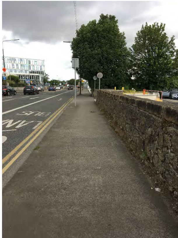
Photograph 1 – View north from leak location
