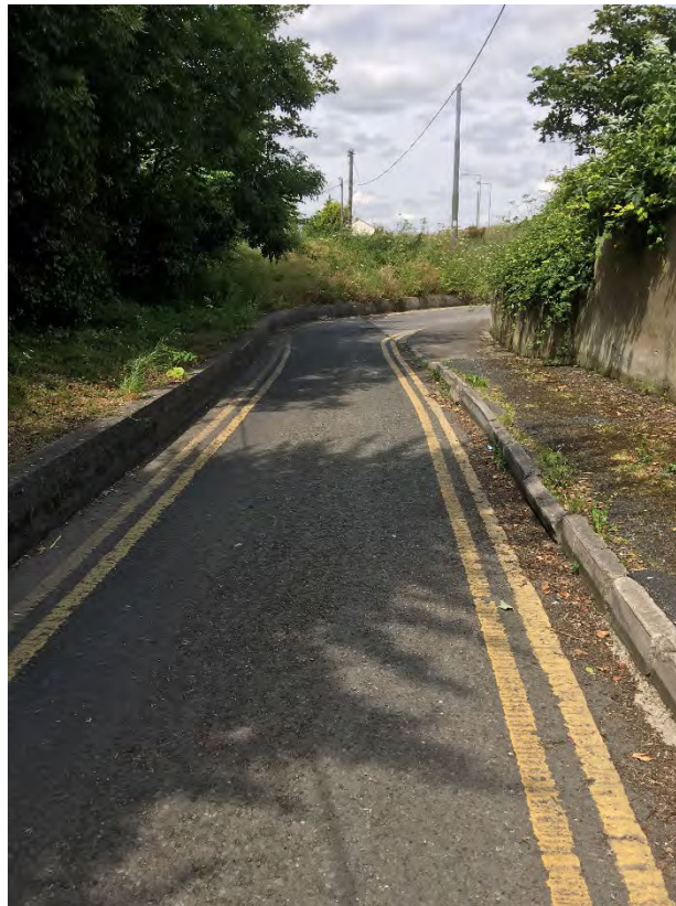
Photograph 4 – View west along Ballyogen Grove
