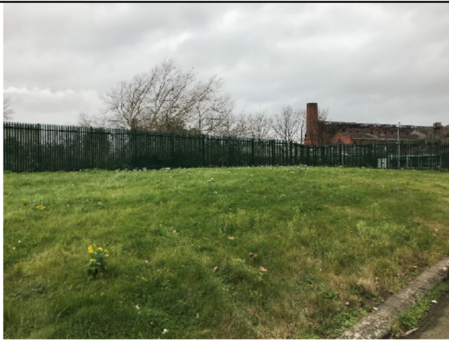
49-01 The cable travels under a green/grassy area at the western most side along the section of interest. No breakout was noted in this area or any other evidence of contamination, (e.g. vegetation die-back, staining, etc.)
