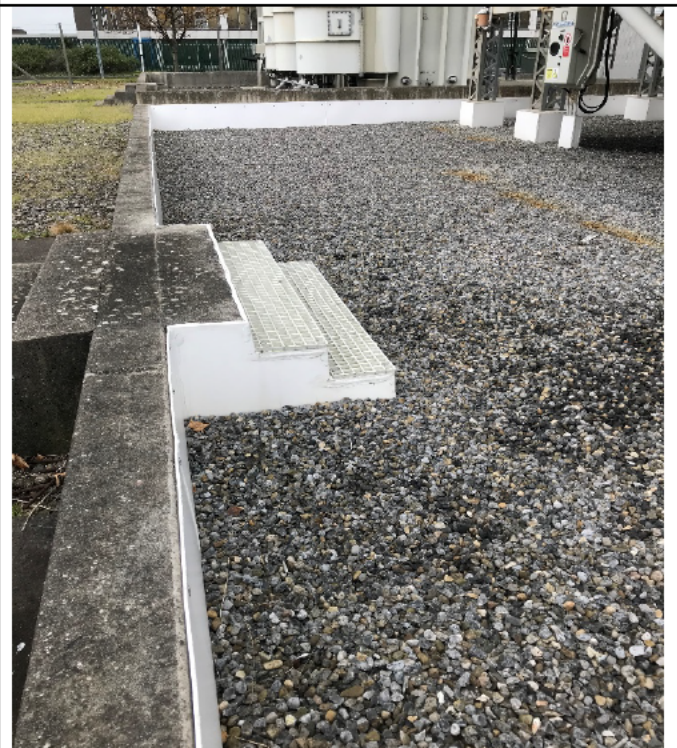
49-04 Recent integrity and relining repairs were evident in this bund
