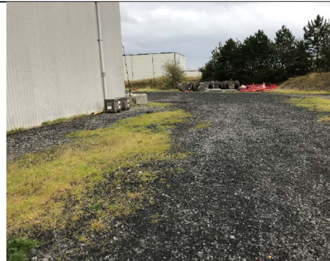
49-07 – The cable travels east under a hardcore surface. As noted, the site representative indicated that the cable under this particular route was removed previously (exact date unknown)
