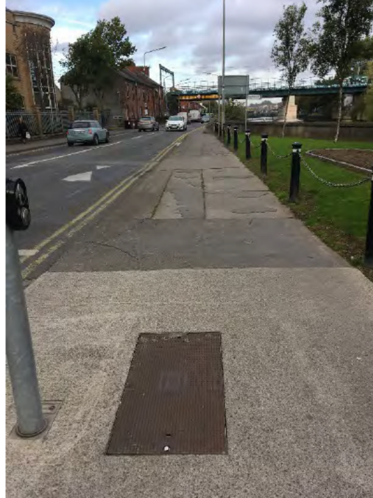
Photograph 3 – Cable route west of leak location
