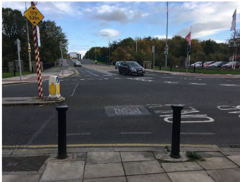
Photograph 1 – Leak location looking north
