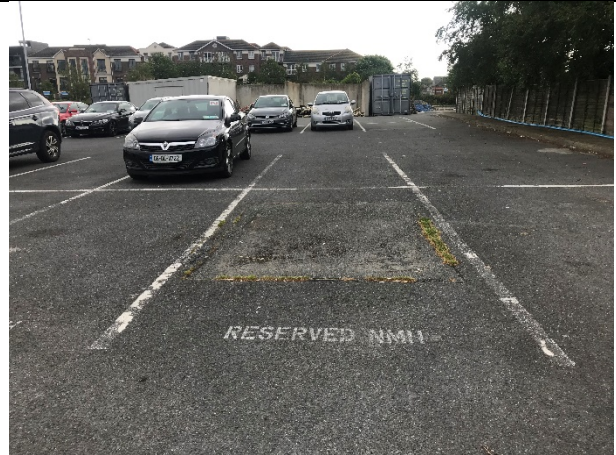
60 –18 – From the mapping it appears that the section of interest turns east after it leaves the ESB networks property. This turn is under the Sportsco access road. The section of interest then runs under a tarmac carpark east towards the River Dodder. The carpark surface was noted to generally be in good condition with only one patch noted in the general vicinity of the cable route.
