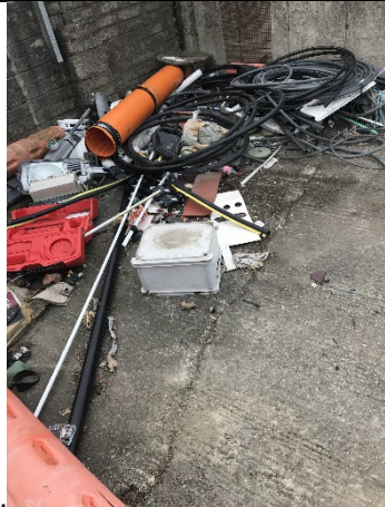
60 –17 – Additional patched concrete base under a waste storage area.
