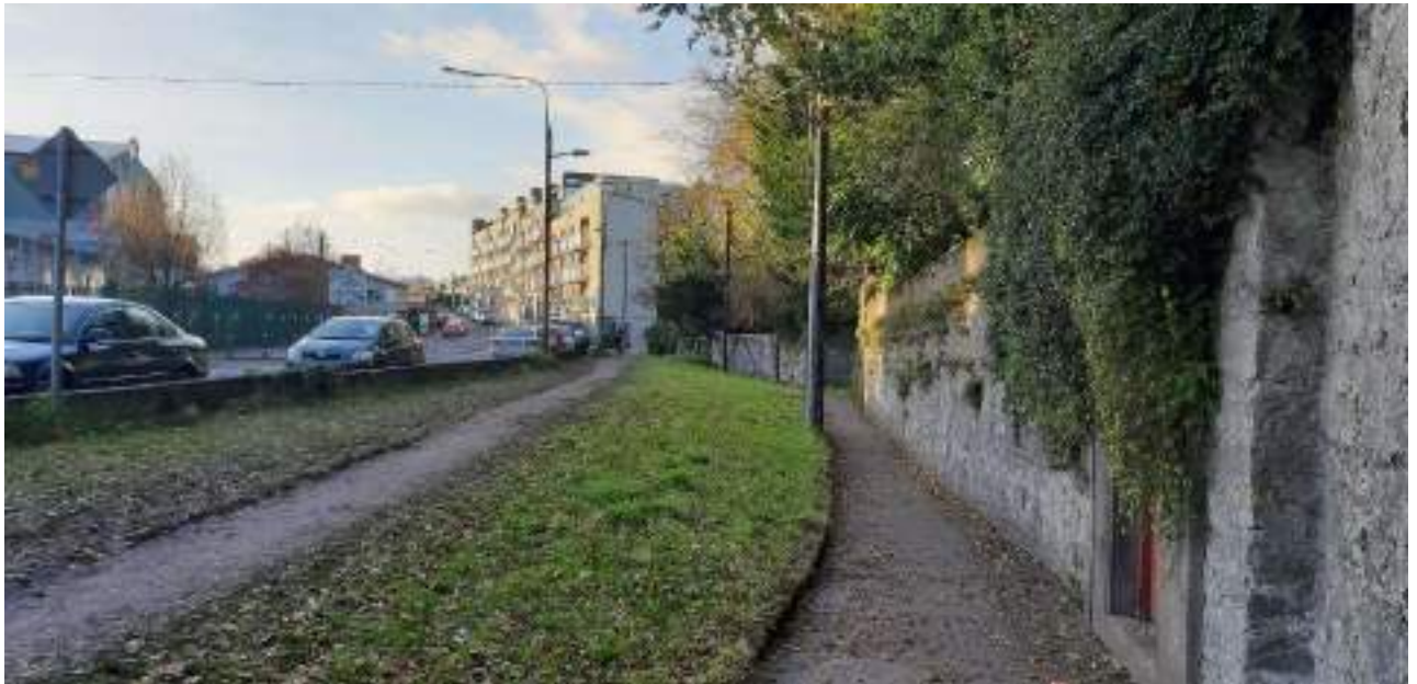
Photo 8. Image, looking west from the area of the leak point, showing the location of the Orchard Gardens apartment complex. Note that the open section of the Glasheen River flows on the north side of the wall seen in the right of this image.
