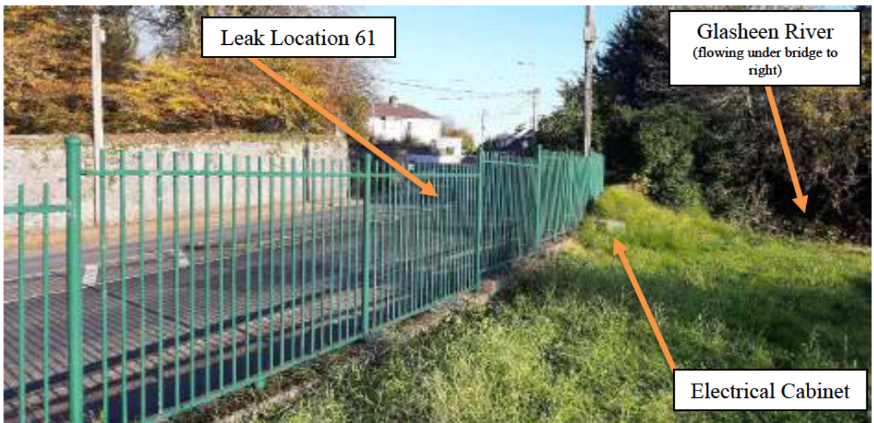
Photo 2. Photo looking east towards indicated location of known leak point (ESB Ref: 61). Note the position of the leak point (background on road); a small electrical cabinet and Glasheen River.
