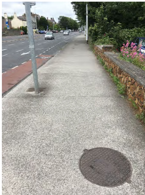
Photograph 6 – View north along Rock Road
