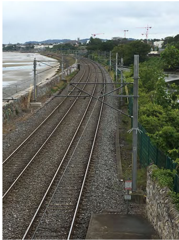
Photograph 2 – View south along cable route
