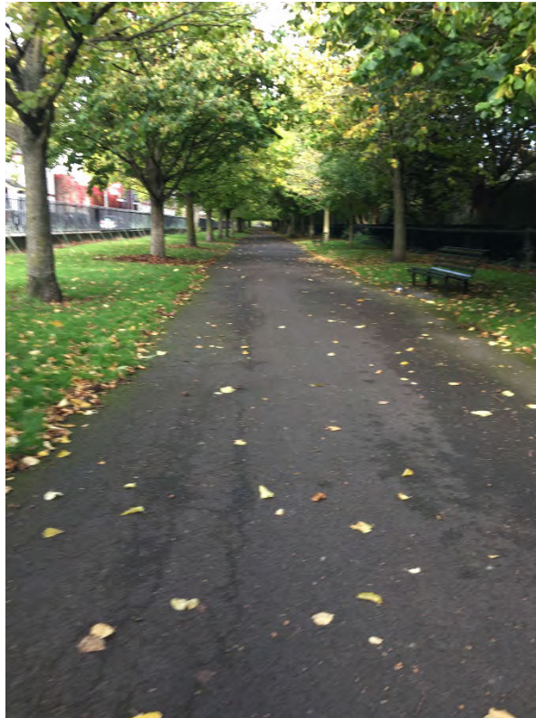
Photograph 1 – Leak location looking north
