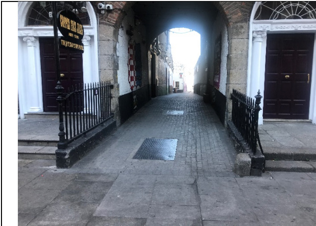
7-01 – Manhole covers present at indicative leak location, at arch to Camden Place.
