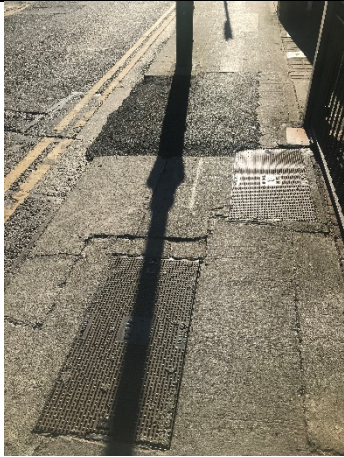
7-13 – Numerous telecommunications conduits noted along the section of interest (Pleasants Street).
