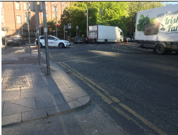
7-07 – Some surface repairs evident on Harcourt Street Upper.
